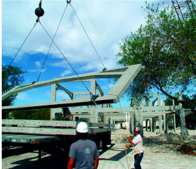
A LadderBlock frame is lifted from the delivery truck.
